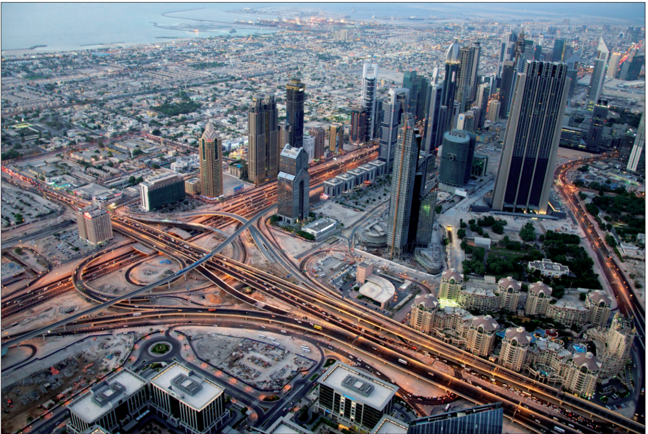
EMIRATI ARABI UNITI-DUBAI, Salini-Impregilo, Dubai Ras Al Khor Crossing
