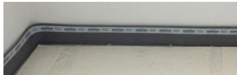
FLEXO is supplied in rolls of 20 cm in height and with a length of 25 m to be applied before the resilient underlay, fixing the gray adhesive strip to the wall in elevation and the white band horizontally, without neglecting the thresholds of the entrances and the doors-windows.
