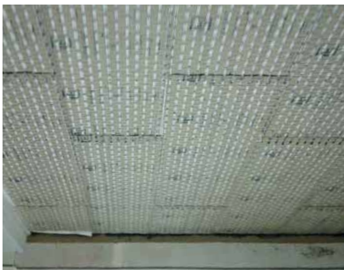
Lastre Stucanet® HBM posate
