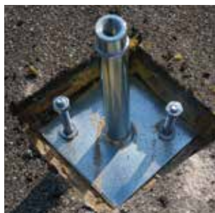
Ritaglio dello strato composto da guaina + isolante e fissaggio piedino Scrap of coating composed by sheath + insulator and fixing foot
